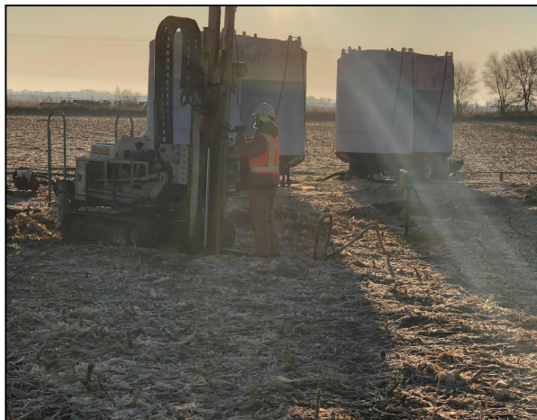
Direct Push rig w/ operator at EW7-T11, points 19-24. 2 x 6,000-gallon trailer tanks w/ mixed amendment in background (facing east)
