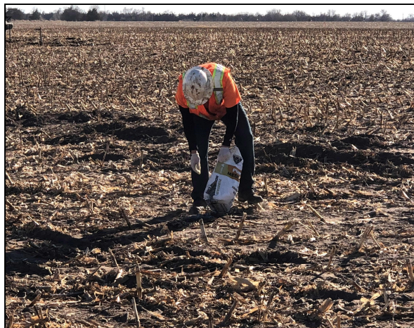
Abandonment of direct push boreholes with hydrated bentonite chips
