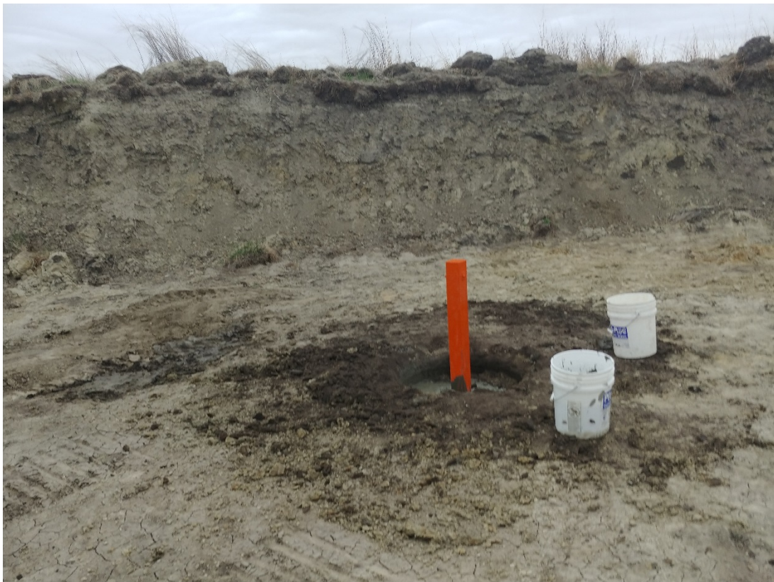
Photo 2 – Installed MW at BKRD-1, near the excavated soil/berm.
