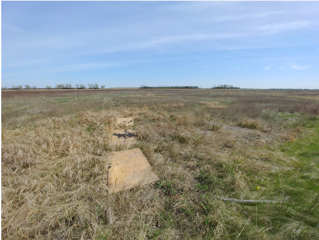
Photo 1 – A “log roll setup using plywood to cross a swampy retention area to the north of Tract 19C to gain access to the UGIA-DPT01 location.
