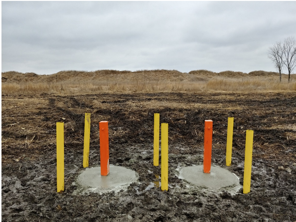
Photograph 1 – Tract 20B MWs 05 and 06 after surface completion; but prior to the permanent placement of the bollards.
