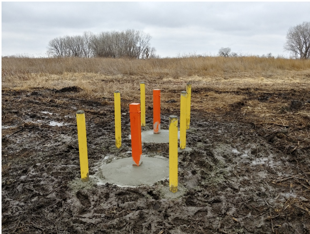
Photograph 2 – Tract 20B MWs 05 and 06 after surface completion and the setting of the bollards.
