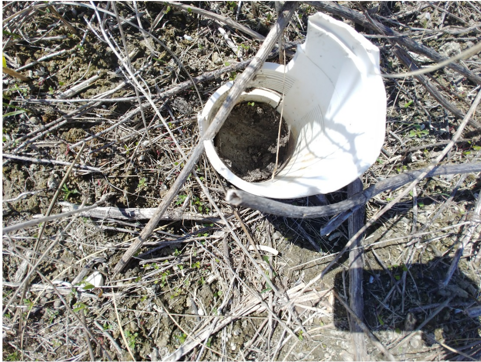
Photo 1 – G0065, at Tract 19C, MW casing packed with hydrated bentonite.
