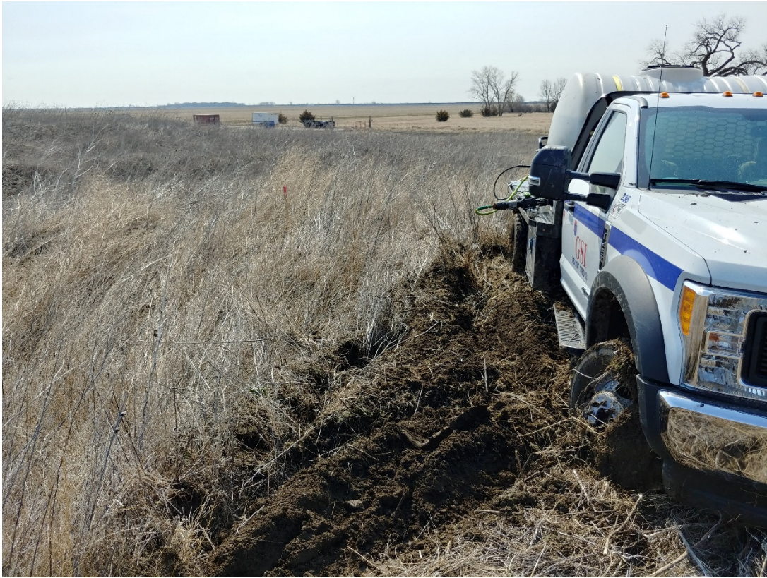
Photo 1 – Soft soil in the Tract 19B stockpile area has made traversing the site difficult.
