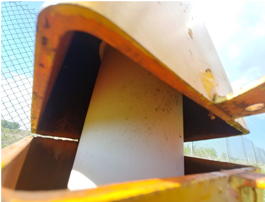
Photo 2 – BGMW01 closeup. PVC casing extended to far into the security lid to allow the lid to be opened.
