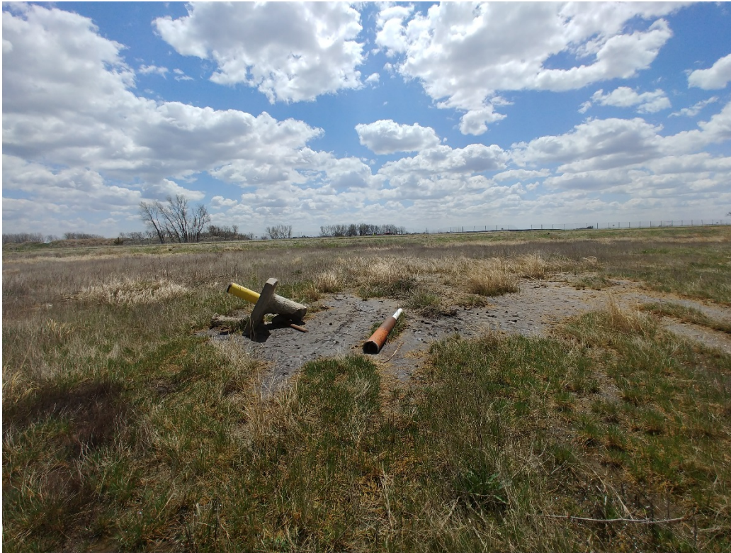
Photo 1 – G0065 (associated with DPT point 19C-UGIA-DPT01) has been improperly abandoned. The remains of the MW were noted during the staking out of sampling locations.
