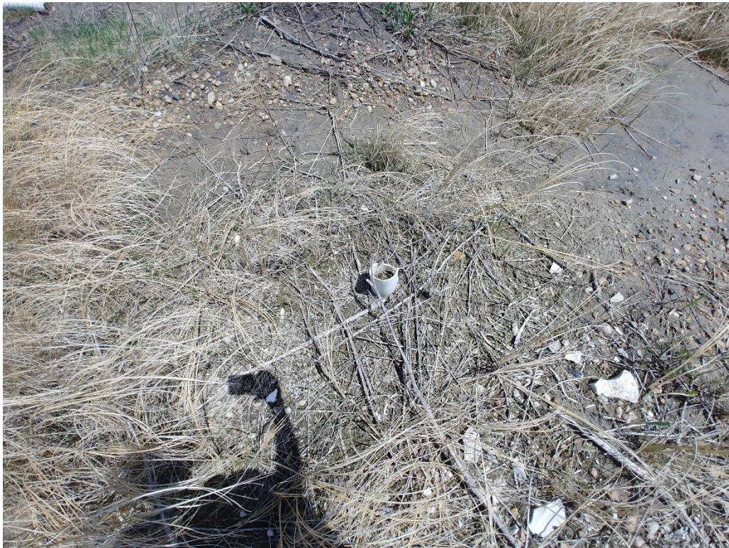
Photo 2 – The well casing of G0065 that marks the remnants of where the well had been installed.
