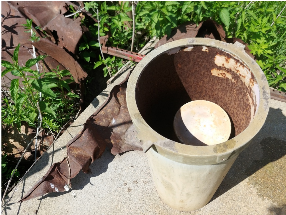
Photo 2- The broken lid on G0071 and intact well cap.
