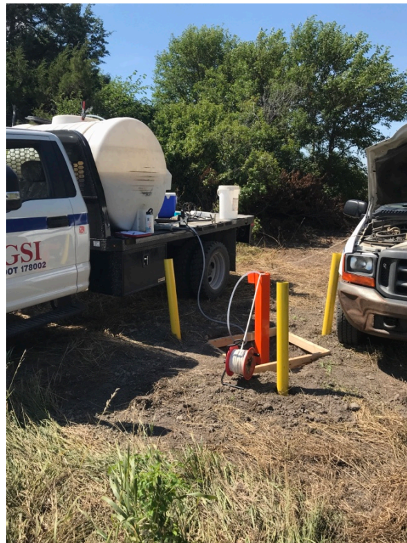
Photo 2: The pad frame is constructed and used to create a square concrete pad. The bollards are also filled with concrete along with the boreholes in which they are installed
