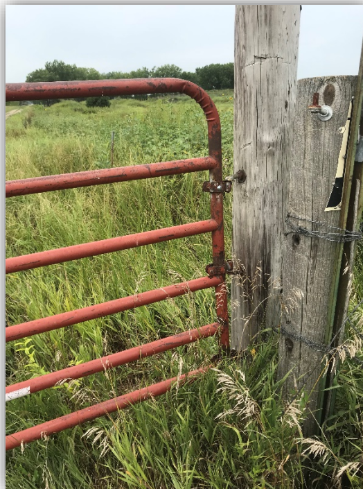
Photo 2: At the intersection of 90 th and Capitol, ATI bolted the upper hinge socket to the gate to prevent dislodging.
