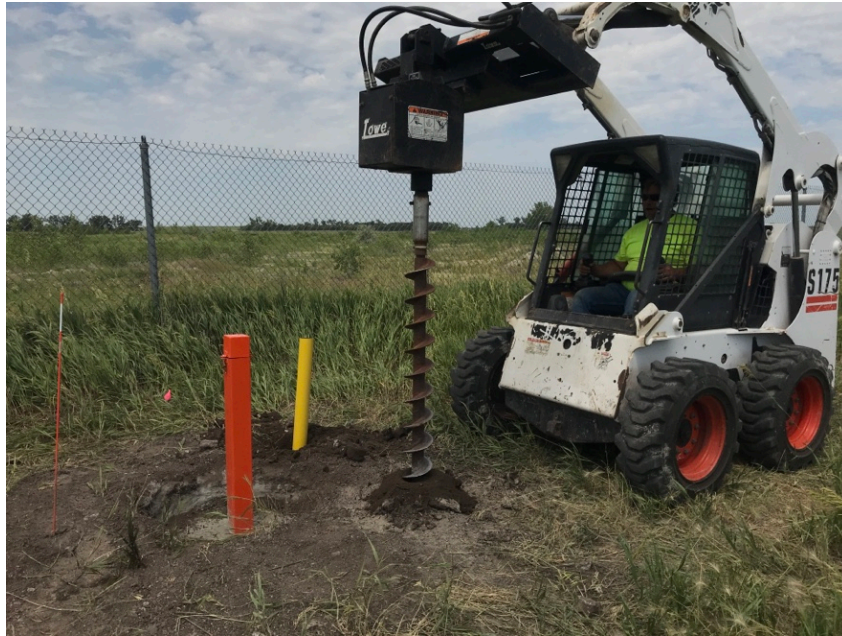
Photo 1: Bollard holes are augered to 2 ft below grade. For efficiency, surface pad and bollard install will occur simultaneously to conserve efforts associated with concrete mixing and application.
