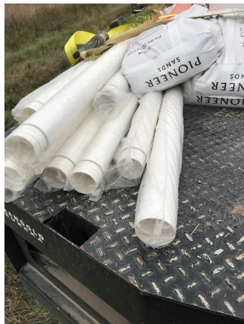
Photo 2: The 2-inch diameter PVC well casing arrives in plastic bags to prevent contamination prior to installation.
