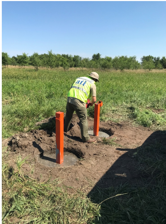
Photo 2: A water level is collected following installation of each well, and is recorded on the boring logs.
