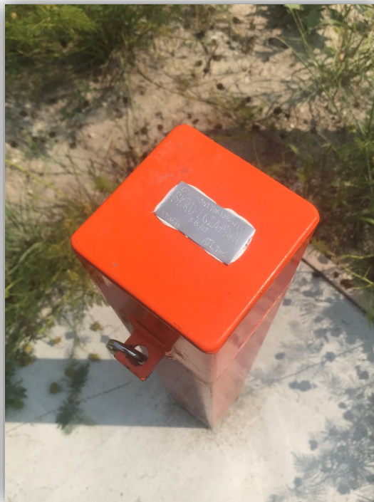
Photo 2: Well details were engraved into aluminum tags that were secured to the well lids using heavy duty glue made for use with painted surfaces, steel, and aluminum.
