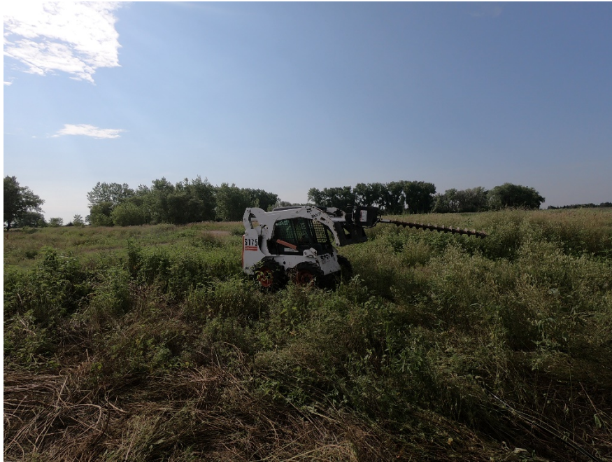
Photo 1: The Bobcat was equipped with an auger that was used to advance the bollard holes.
