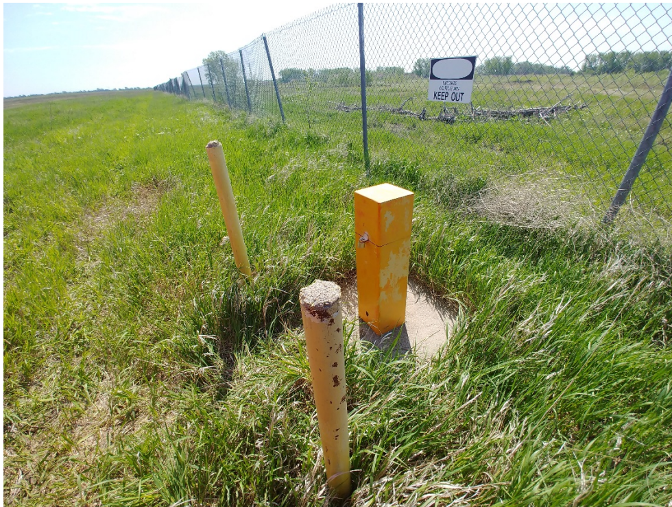
Photo 3 – BGMW01 after .56' of PVC was removed from casing.
