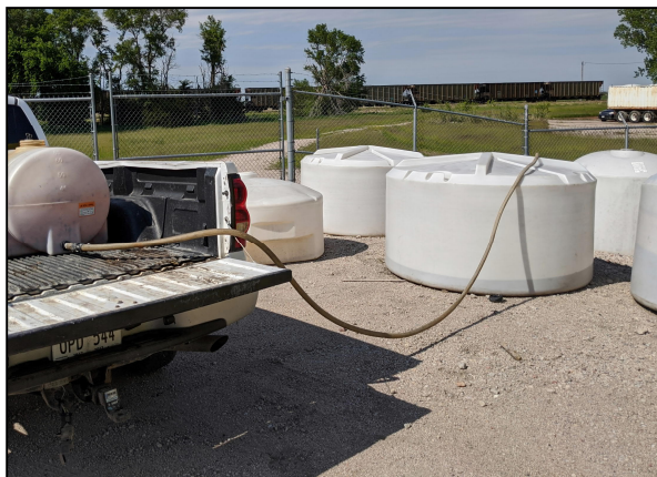
Purge and decon water transfer to IDW tank at GWTF (facing north).
