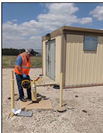
Water level measurements at extraction well 5 observation wells (facing north).
