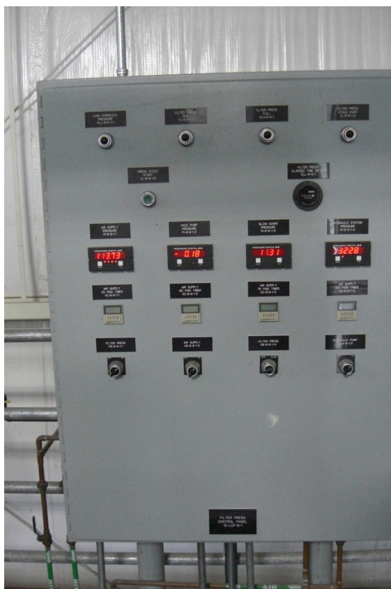
Photo 12 Date: July 31, 2014 Site: CHAAP Description: Filter Press Control Panel in GWTP.
