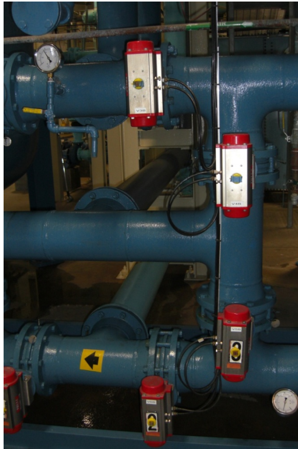
Photo 5 Date: July 31, 2014 Site: CHAAP Description: GAC Air Actuator Valves in GWTP
