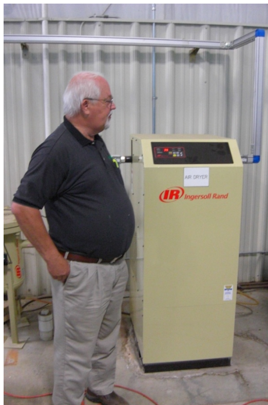
Photo 6 Date: July 31, 2014 Site: CHAAP Description: New Air Dryer in GWTP
