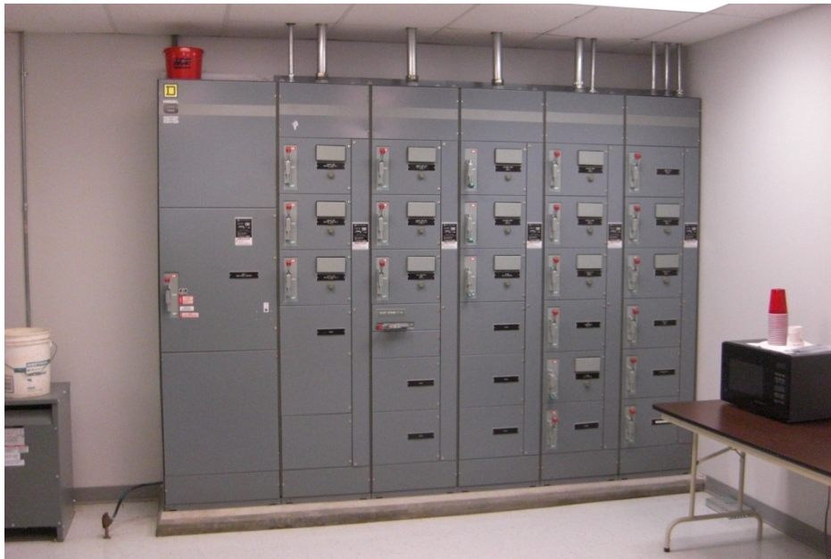
Photo 17 Date: July 31, 2014 Site: CHAAP Description: Motor Control Center – main electrical panel in GWTP.
