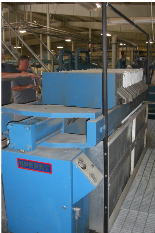
Photo 11 Date: July 31, 2014 Site: CHAAP Description: Filter Press in GWTP.
