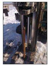
Installation of temporary PM wells: EW7-PM26A (shallow) and PM26B (shallow intermediate)
