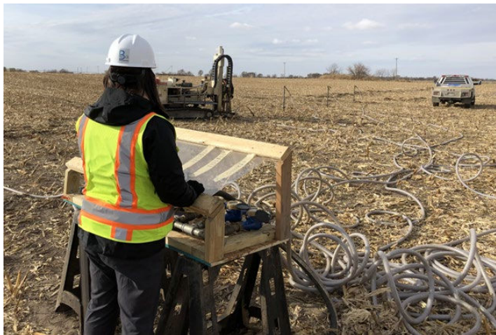
Subsurface injection of amendments into the aquifer.
